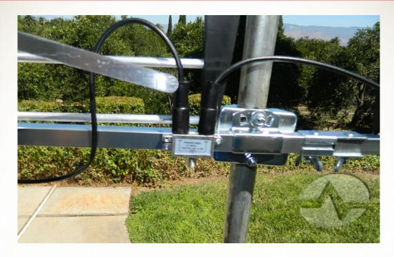
Turn the assembly right side up so you can see the cables and the combiner
