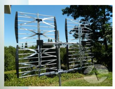
As you look at the antenna, you will see that the mounting point has an adjustment to help you keep the antenna pointed properly. In most cases this should not be used. Instead, level and plumb the mast properly.
